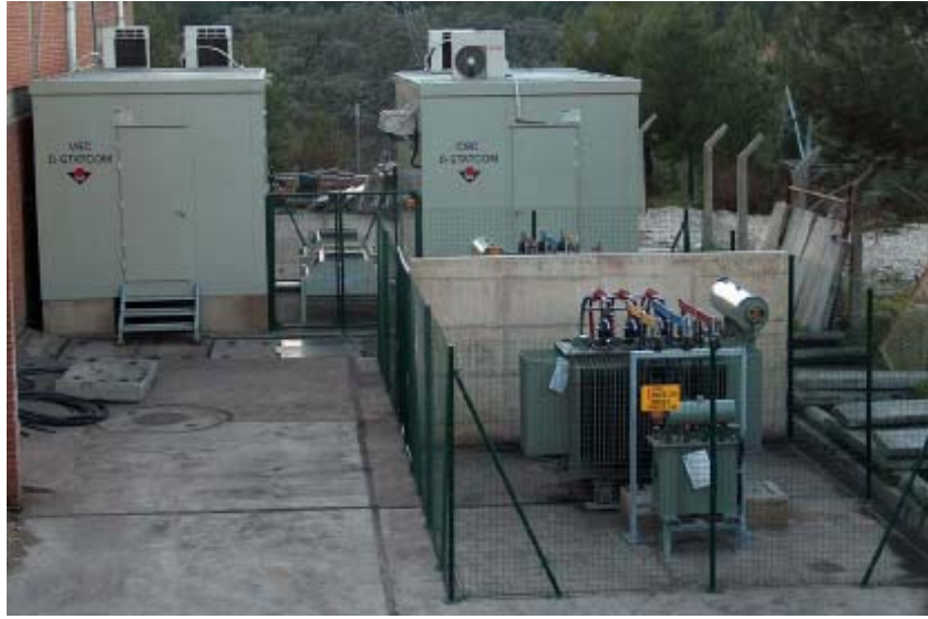
Fig.1.5. VSC and CSC STATCOM systems in KEAŞ, Turkey
