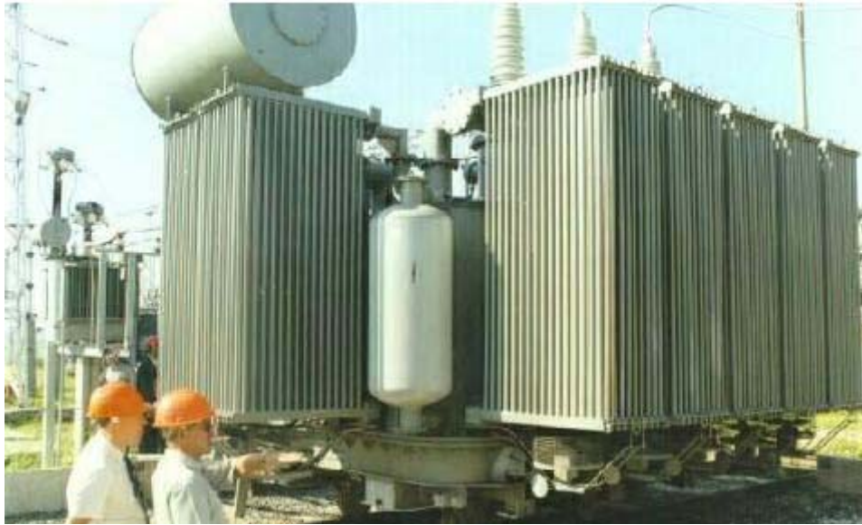
Fig.1.2. 25MVA 110kV shunt magnetically controlled (Saturated) reactor connected to 32MVA Capacitor bank, installed in Kudymar Substation, Russia. [65]
