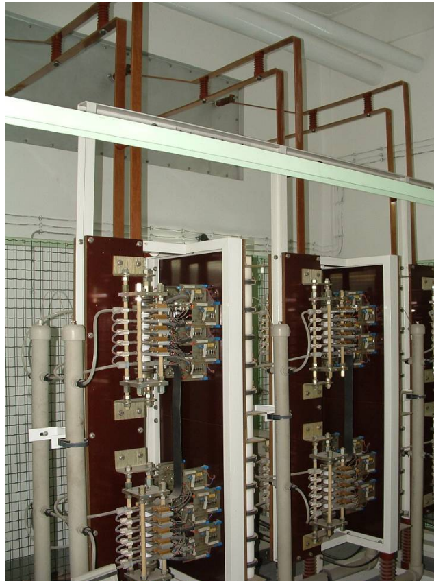
Fig.3.6. A series operation of back to back three phase thyristor stack configuration
