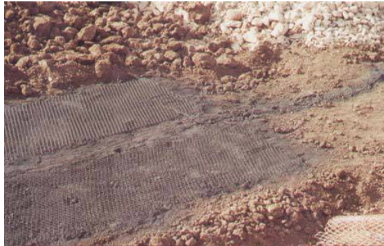
Fig.4.24. Ineffective attempts to reduce ground resistance for surface limestone sites
