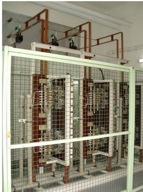
Fig. 5.23. Power stage of 6-pulse TCR-2
