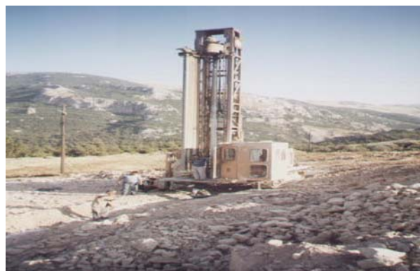
Fig.4.23. Drilling holes for grounding rods
