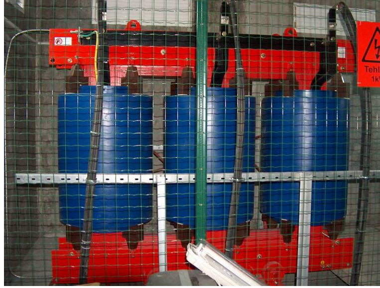
Fig.1.3. Reactors of a Y-connected TSR installed for Bursaray, Turkey for the compensation of underground cables installed for light railway.
