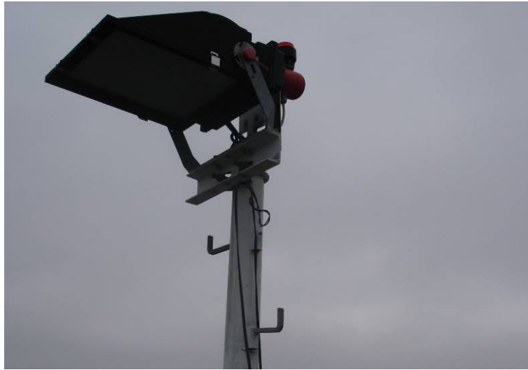
Fig.4.17. Audio-visual alarm systems, red-flashing light and an audible alarm mounted right at the bottom of it on the light post.
