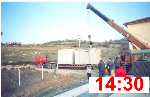
Fig.4.56. Step by step relocation of the SVC system in TKİ Bİİ because of the landslide (a-h).
