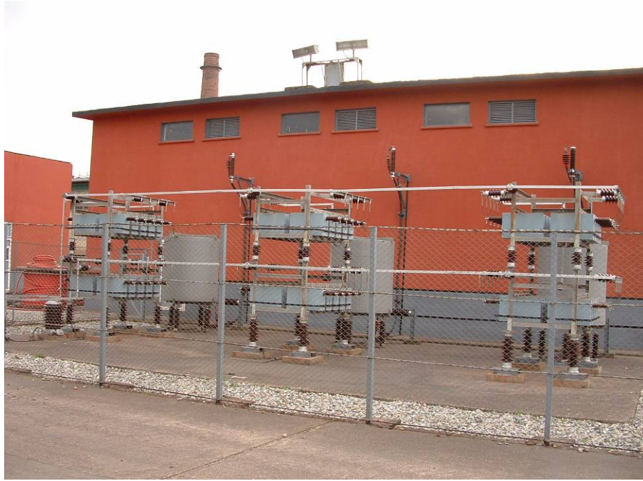
Fig.5.4. Existing 13 MVar 3 rd Harmonic filter of LF.
