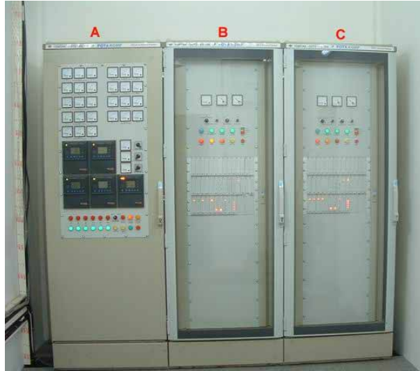
Fig.5.22. (A) Protection and monitoring panel, (B) Control panel for TCR-1 and (C) Control panel for TCR-2 (If one is chosen as the master control unit the other can act as the slave)
