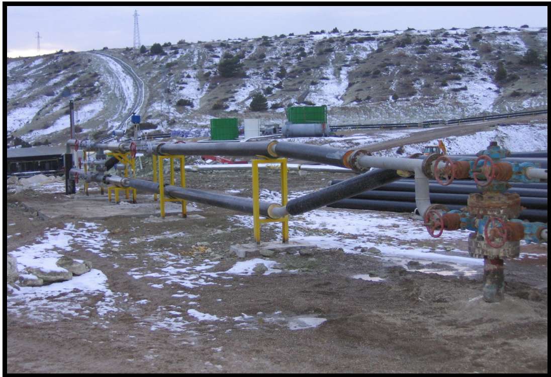
Figure 4.9 Constructed well head and pipeline
