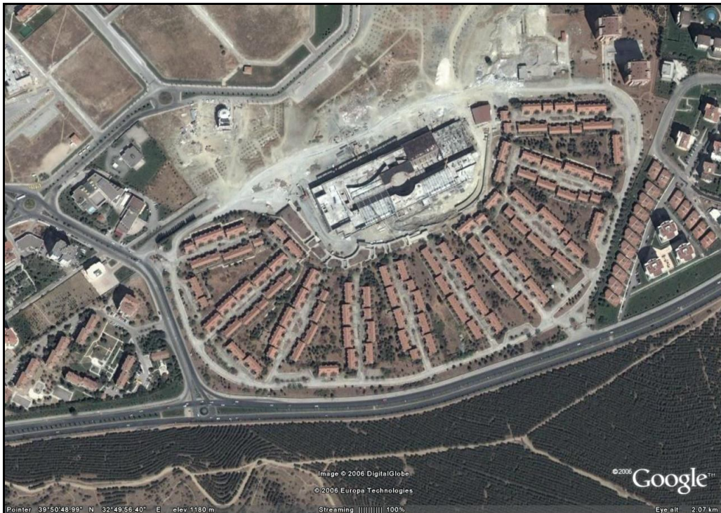
Figure 8 An aerial view from the shopping mall on construction and deputy residences by Google Earth.
