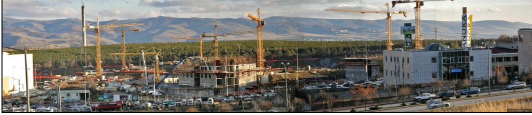
Figure 11 A photo of the construction of Park Oran Konutları .
