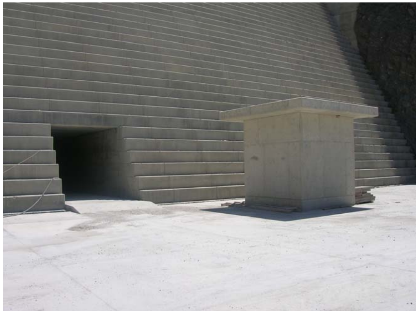
Figure 4.13. Automatic Data Acquisition System House located at the 220.50 m elevation downstream
