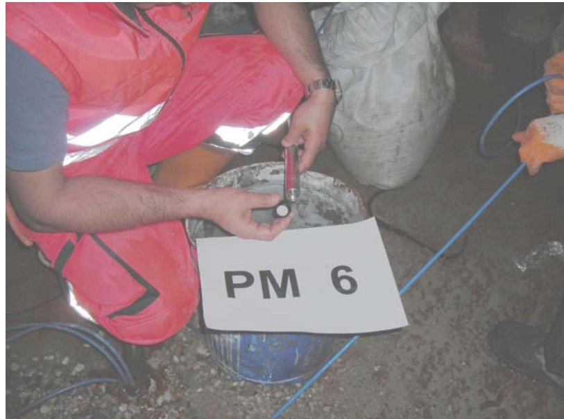
Figure 4.1. Installation of PM6 labeled VW piezometer at Cindere Dam
