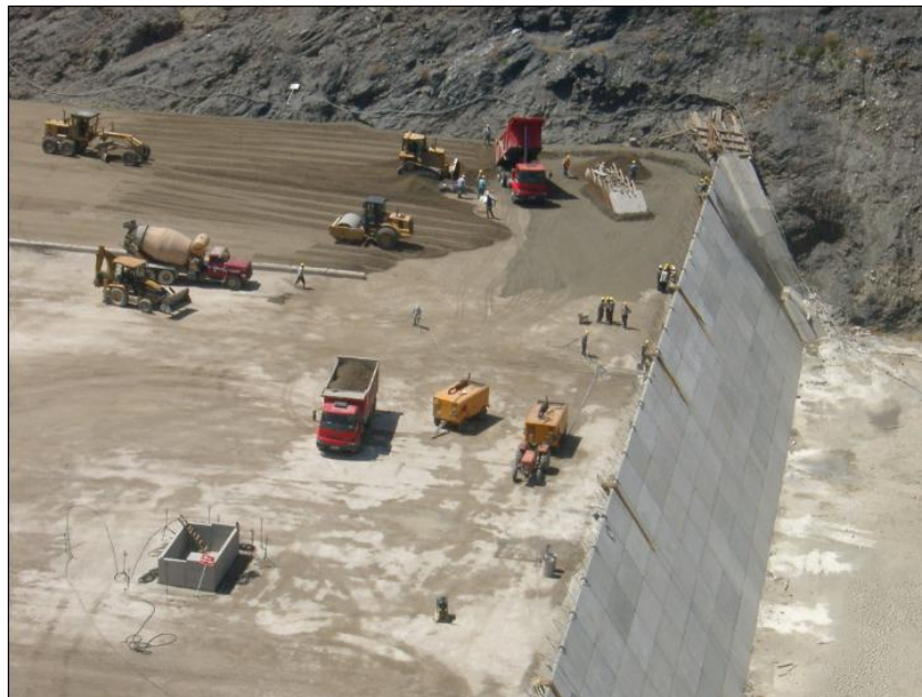
Figure 1.1. A photo taken during construction of Cindere Dam (Gürdil, 2003)
