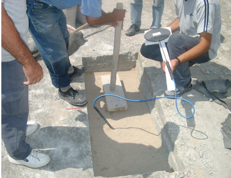
Figure 4.4. Installation of a VW pressure cell at Cindere Dam
