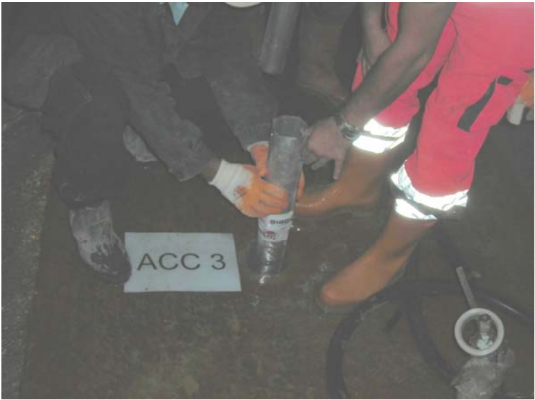
Figure 4.10. Installation of accelerometer tube at Cindere Dam
