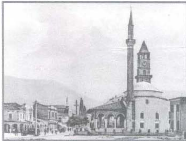
Figure 5: View of Ethem Bey Mosque (B. Aliaj, K. Lulo and G. Myftiu, Tirana the Challenge of Urban Development, p.19)
