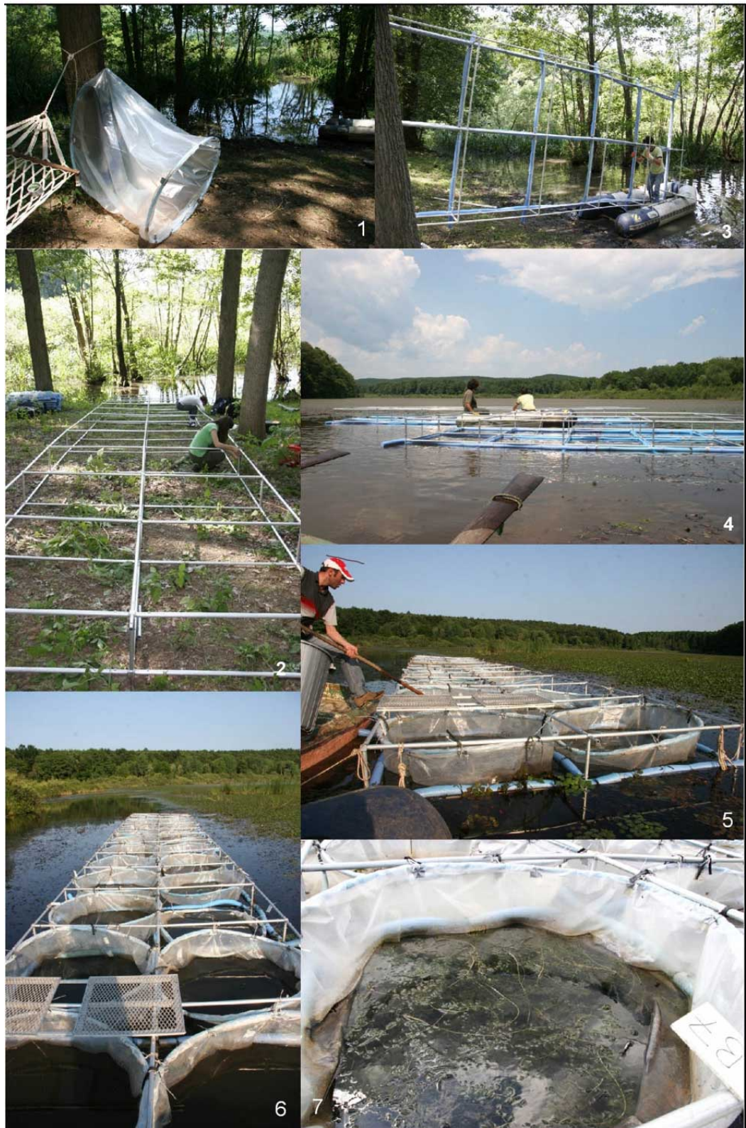
Figure 2.3: Sequences in the construction of the mesocosm .
