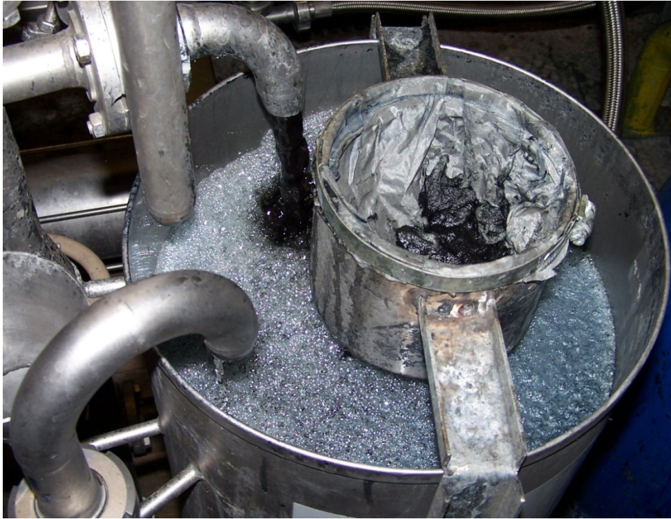
Figure 4.16 SelRO MPT-34 Pilot system feeding tank coarse filtration unit
