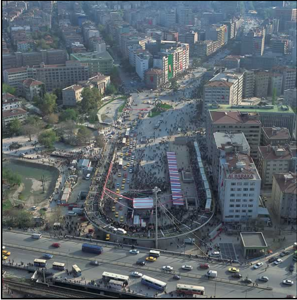
Picture 50. Sıhhiye Square and the Sıhhiye U-Turn in 2005 Source: The page of Yapı Proje Merkezi http://www.ypm.com.tr
