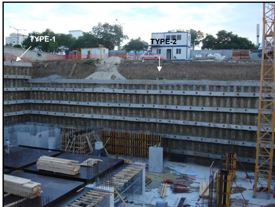
Figure 140. Views of the site
