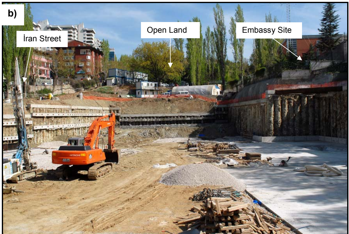
Figure 119. Views of the site
