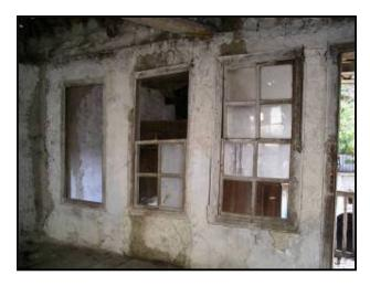
**Figure 80:** The Missing Door and Window Wing at FF06 Space (author April, 2003)
