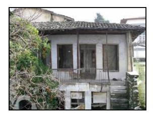
**Figure 79:** The Missing Door and Window Wing at First Floor (author April, 2003)
