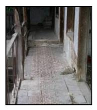
**Figure 55:** The Level Difference on the First Floor of South-east Mass (author April, 2003)
