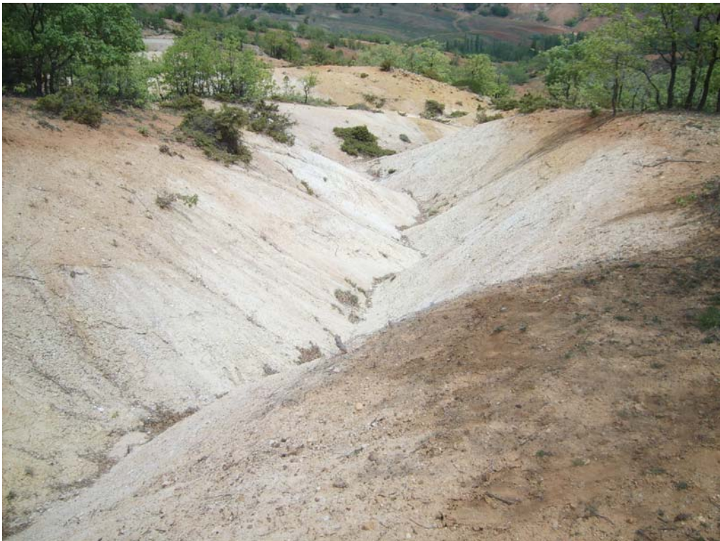
Figure 5.5. Photo from the location 4.
