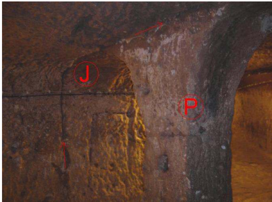
Figure 5.26. Joint juxtapose to the pillar in 4 th room of Derinkuyu. (J: Joint, P: Pillar)
