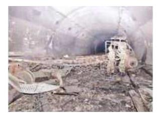
Figure 2.1 Large Extreme Tunnel Fire (Trucks Carrying Missiles Caught Fire and Melted, No Signs of Concrete Spalling), South Korea: November 2005
