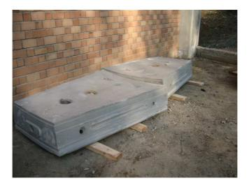
Figure 3.1 Precast TBM Key Segments
