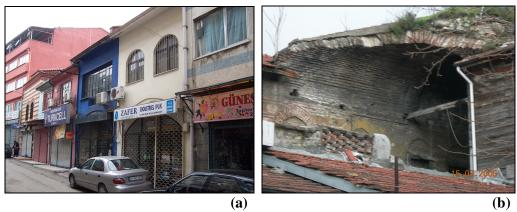
**Figure 2. 50 : (a)** Five small units of Y.G.P.H. at the south of Cumhuriyet Street **(b)** partially collapsed vault at the PART I of Y.G.P.H.
