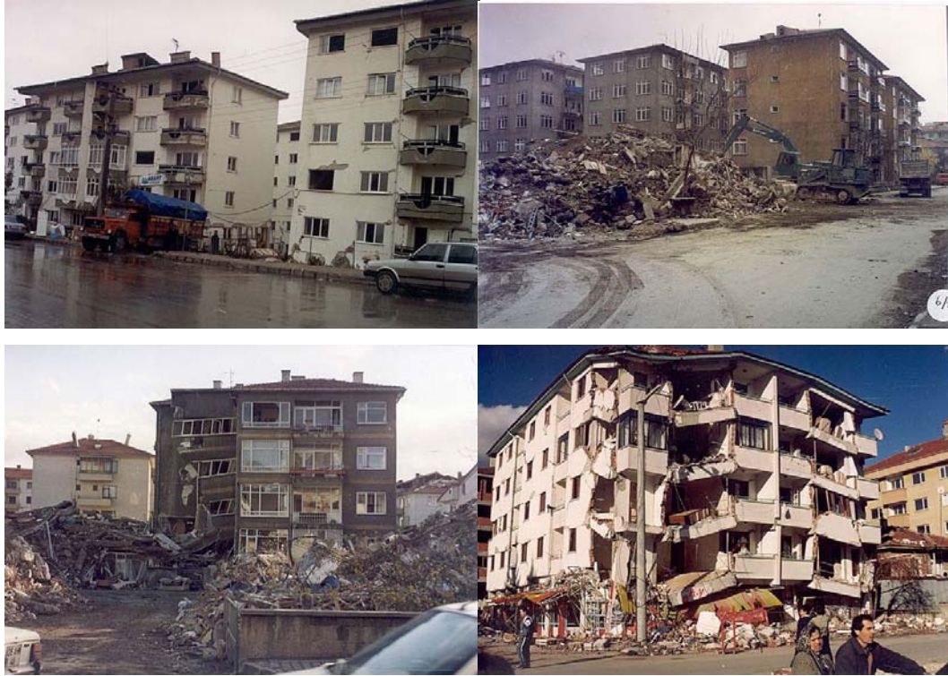
Figure 2.7 Buildings Damaged in 1999 Earthquakes in Bolu
