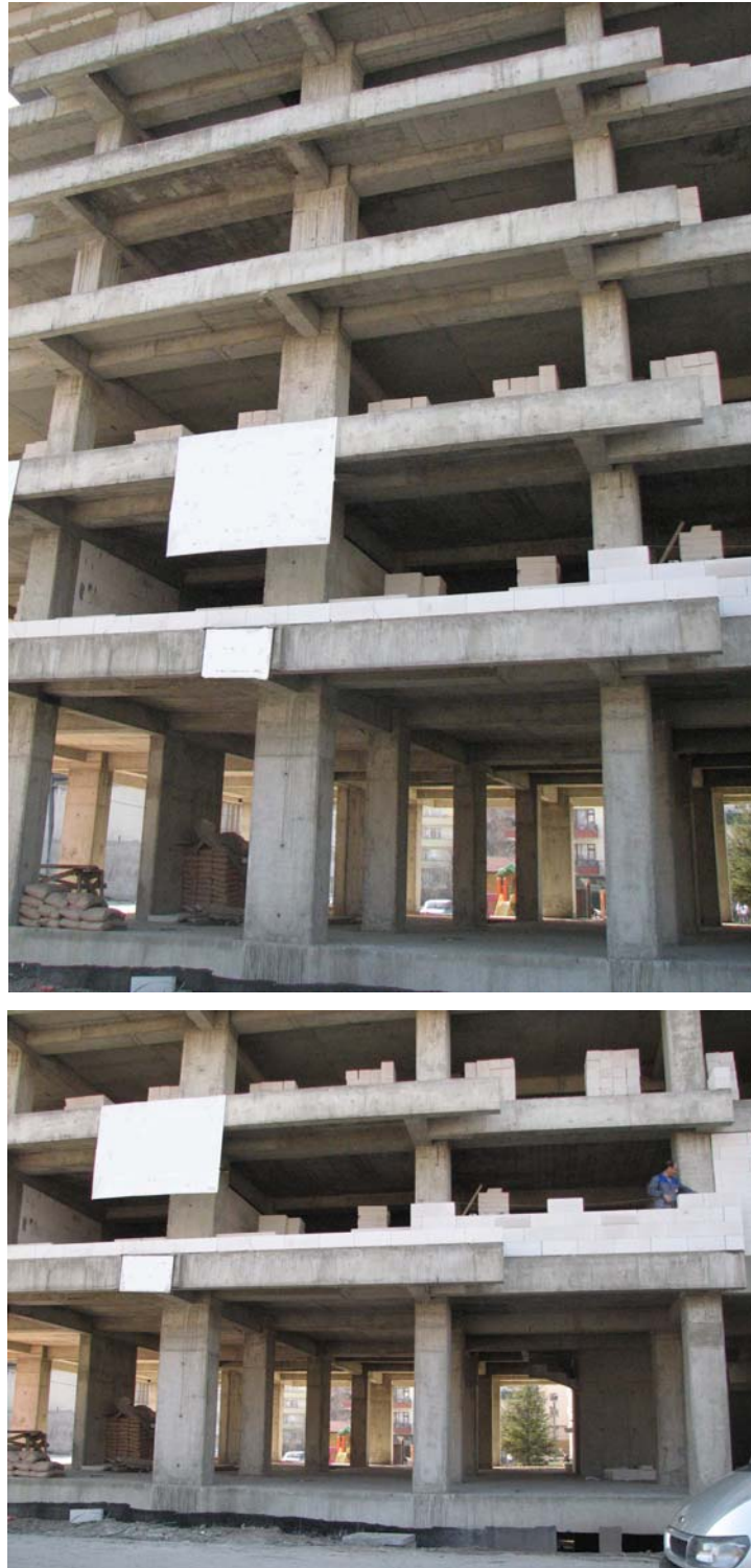
Figure 6.3 A Building Construction in Bolu with Regular Structural System 2008
