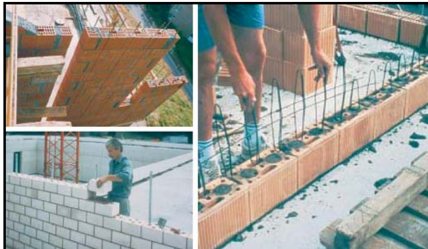
Figure 2.15 Reinforced Masonry Wall Construction (Bachmann, 2003, pp.34-35)
