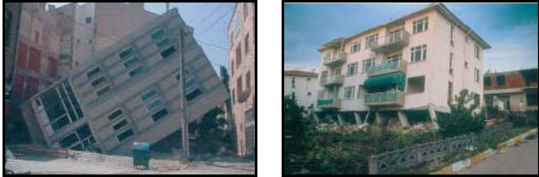
Figure 4.4 (Continue) Heavy Damages of 1999 Earthquakes in Turkey (Bachmann, 2003, pp. 15, 67)
