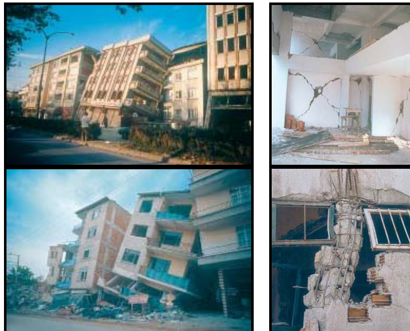
Figure 4.4 Heavy Damages of 1999 Earthquakes in Turkey (Bachmann, 2003, pp.15,20,31,45,66)
