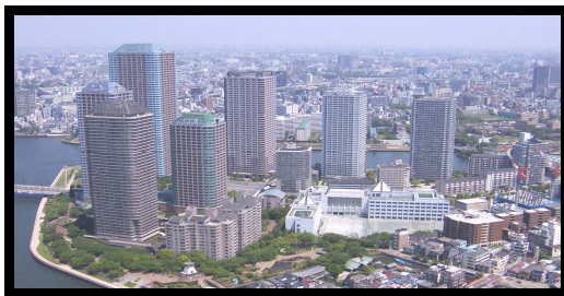
Figure 2.19: Okawabata River New Center Dome (Chuo Ward, Tokyo) (Gökçe, 2007, pers. archive)
