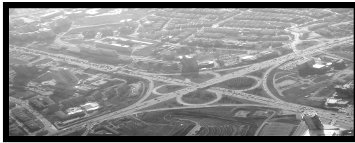
Figure 4.38.: Konya-Eskişehir Roads Intersection (wowturkey, 2008)
