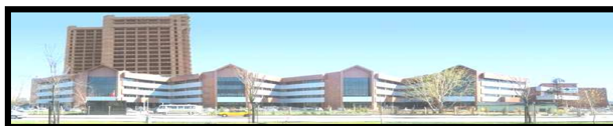
Figure 4.37: A Landscape from Söğütözü-Media Center (wowturkey, 2008)
