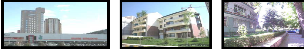
Figure 4.45.: Office Buildings; Çayyolu-Mesa, Beysukent, Mebusevleri (wowturkey, 2008)
