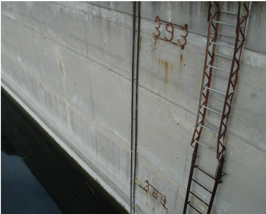
Figure 4.11 Reservoir level measurement
