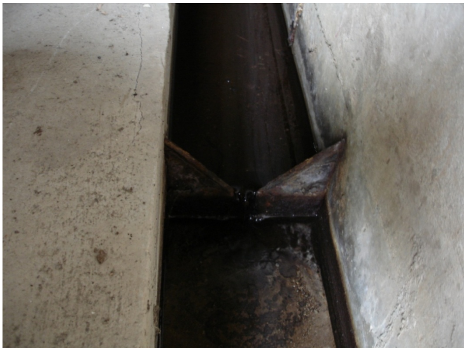
Figure 4.14 Triangular weir (B-18)
