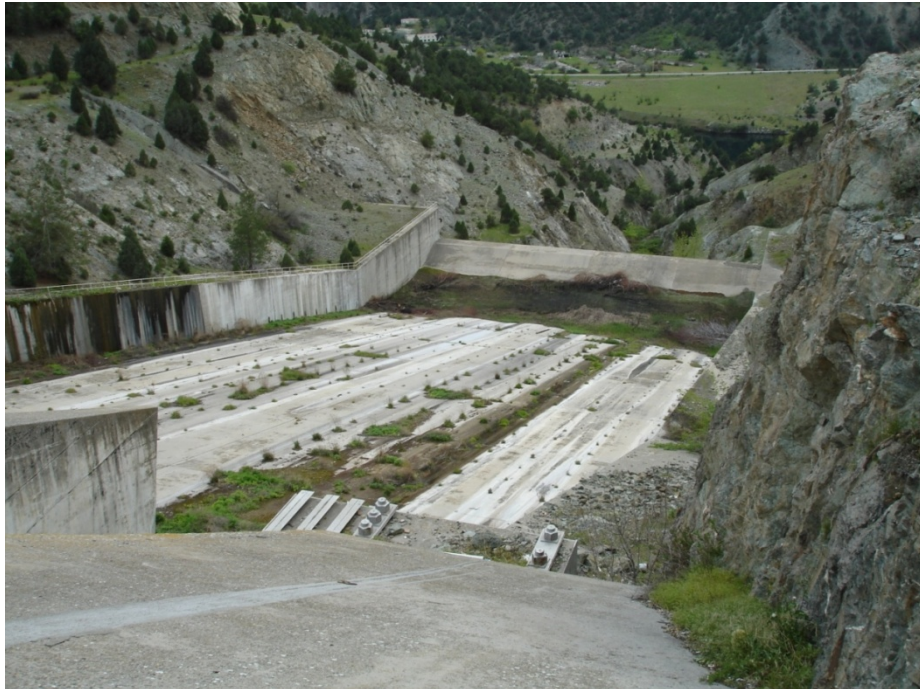
Figure 4.24 Gökçekaya Dam Spillway
