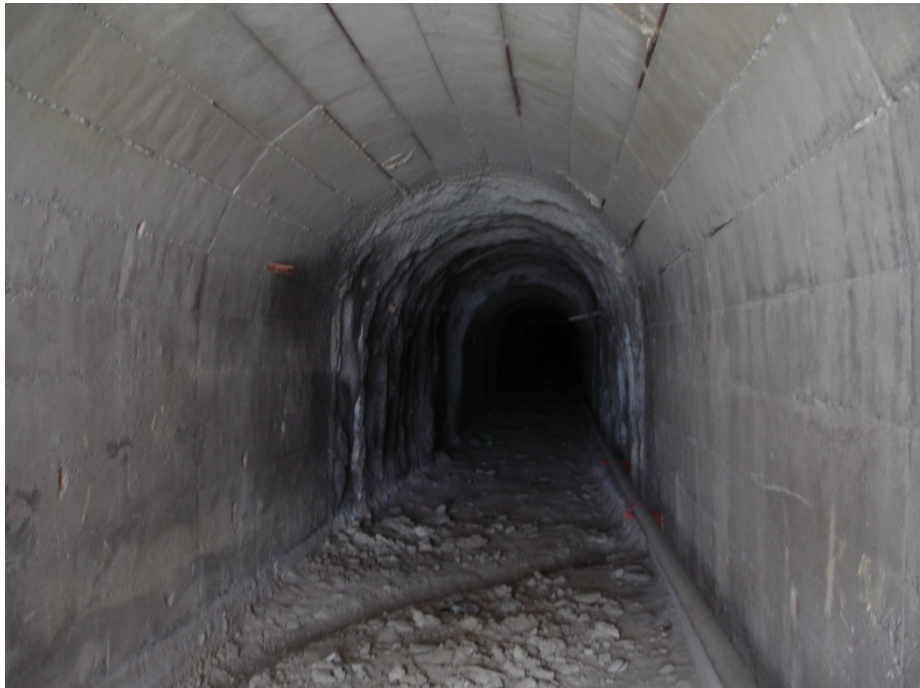
Figure 4.7 Left abutment inspection gallery (LA-1)
