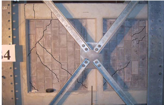
Figure 5.35 - Cracking on the Infill in the Six Cycle
