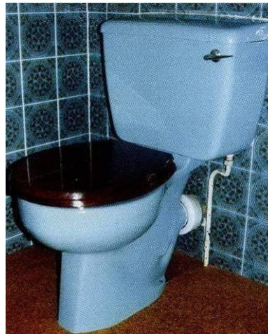
Figure 2.45 Double Trap Syphonic WC Suite (Blair, 2000).
