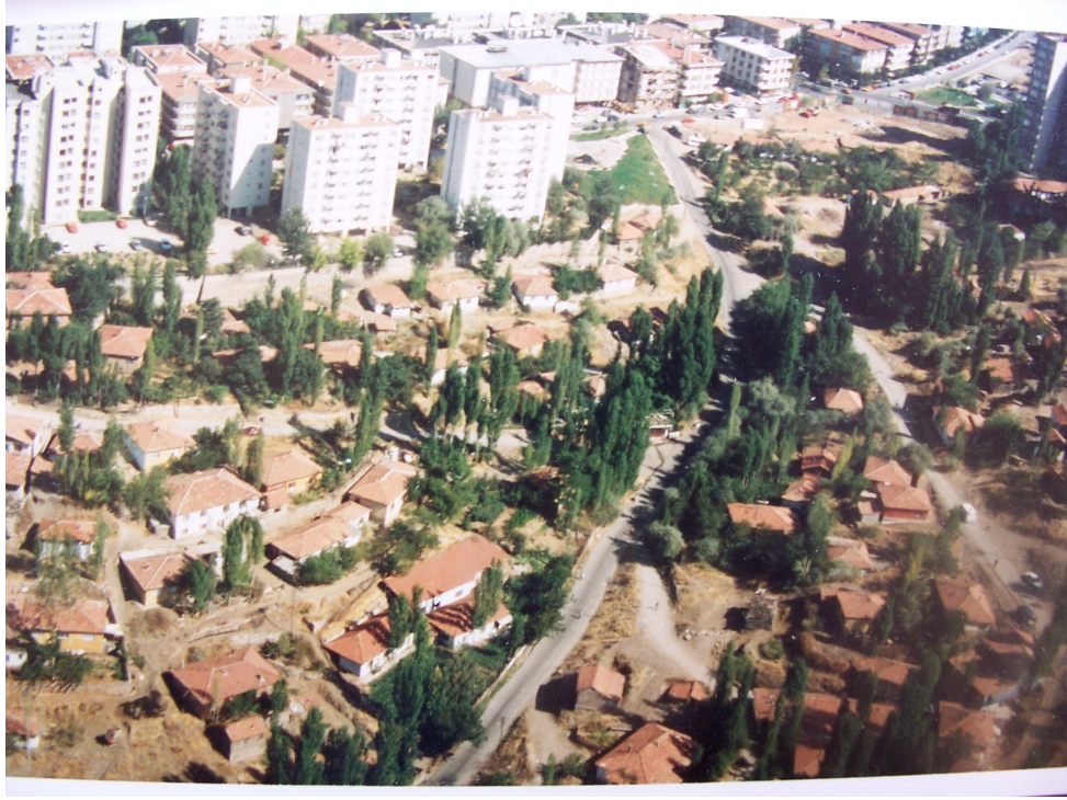
Figure 7 Inadequate living conditions in the Dikmen Valley
