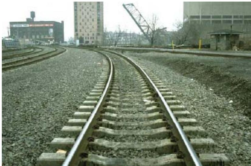
Figure 4.8: Preview of a track with concrete tie
