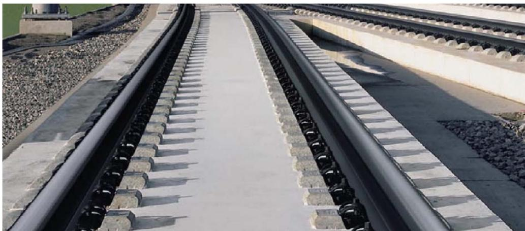
Figure 4.6: Direct fixation track on segregated open area
