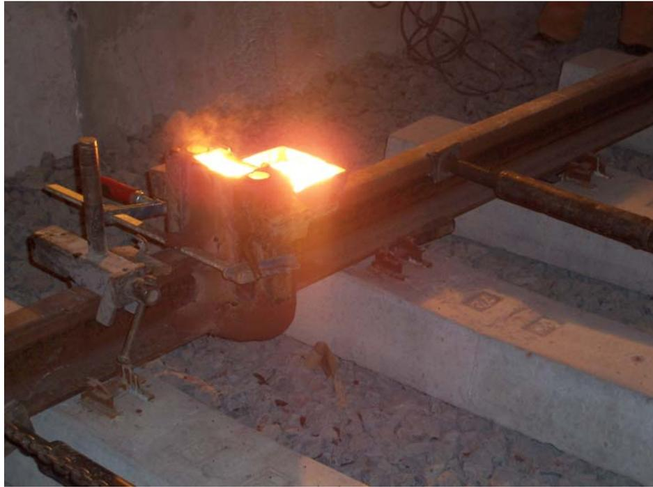
Figure 4.11: Thermite welding application photo taken by Öztürk.E
