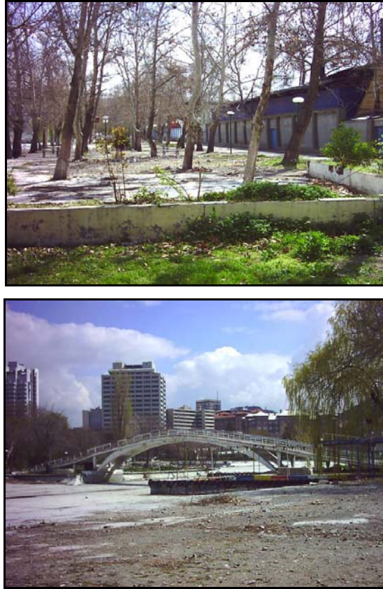
Figure 4.31 Photos of the Demolition Progress (Author, 16.04.2007)
