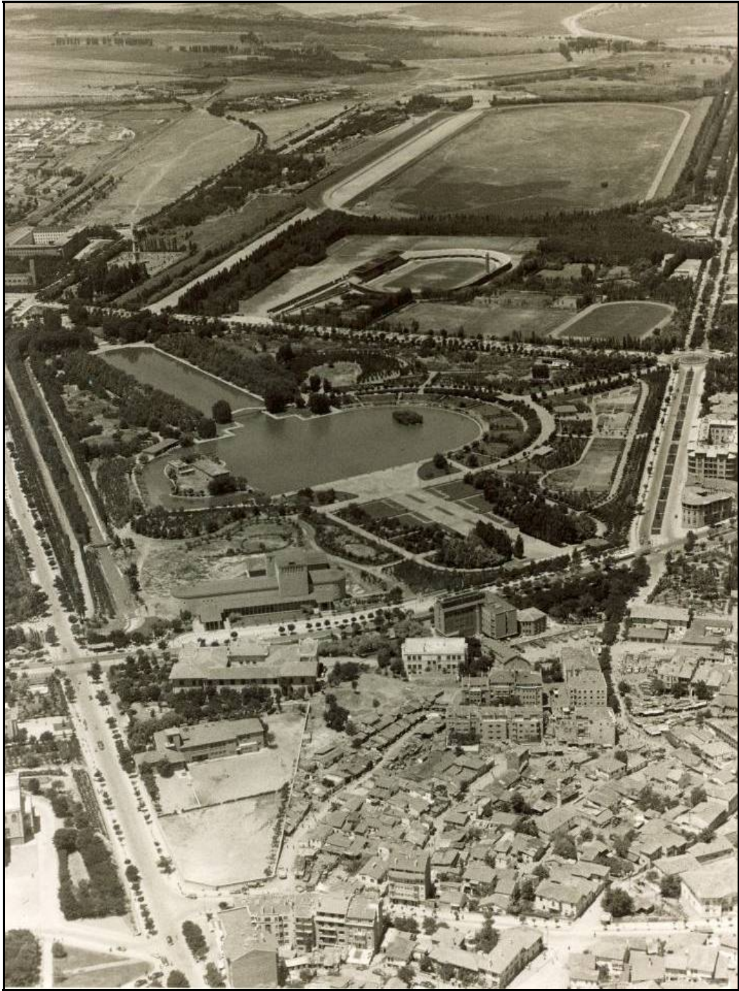
Figure 4.1 The Aerial View of Gençlik Parkı, 1953 (VEKAM, Photograph and Postcard Archive, no. 523)
