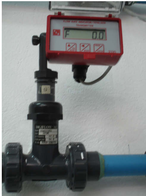
Figure 2.3 Turbine Type Flowmeter
