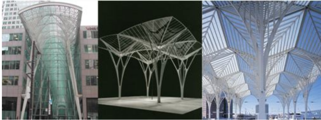
Figure 3.4 Examples from Calatrava's tree-like structures BCE Place, Bauschanzi Restaurant Oriente Station (Source: Zardini, 1996)
