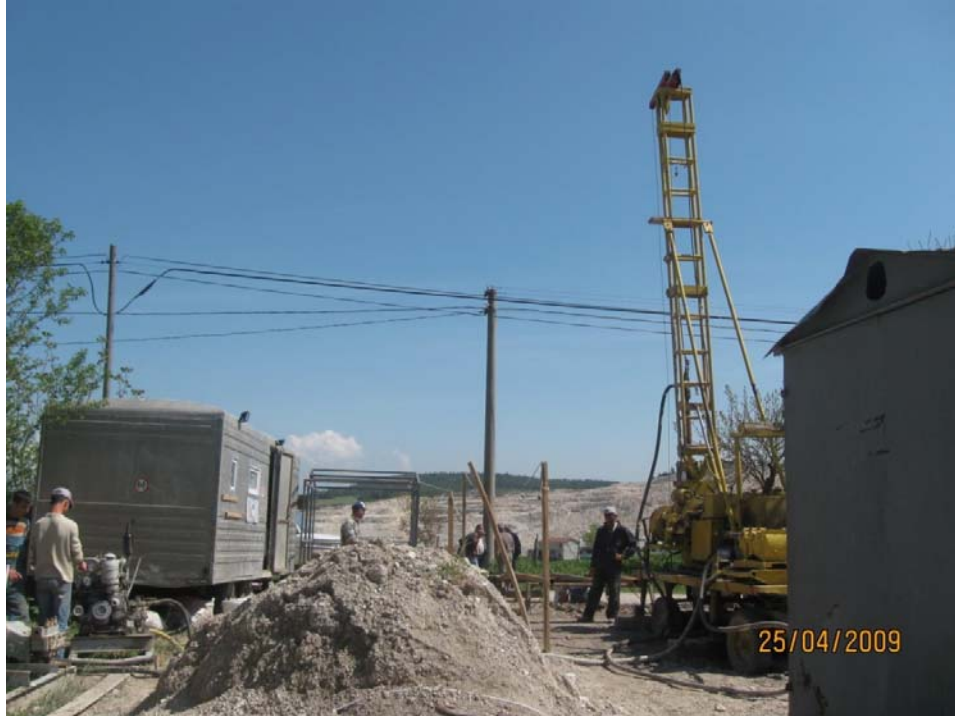
Figure 3.9 View from Drilling of MTA nearby Tulu Mine
