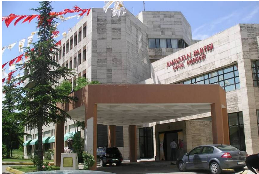
Figure 4.8: ANAP Headquarters: view towards the main entrance
