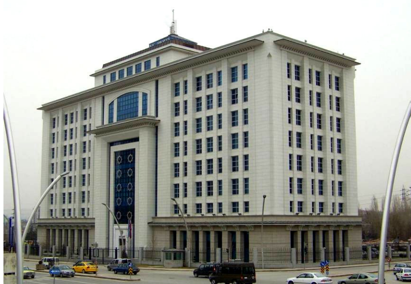
Figure 4.2: AKP headquarters: the entrance emphasizing the presidential floors
