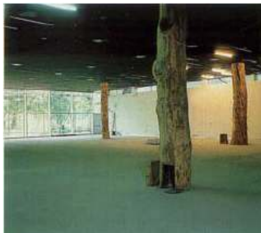
Figure 3.19. Tree-trunk columns of the lower hall of the Kunsthall. Source: DaapSpace Website. Retrieved May 05, 2009 from ( http://www.daapSpace.daap.uc.edu/~larsongr/Larsonline/Koolhaas_files/Oma.Kunst.pdf )
