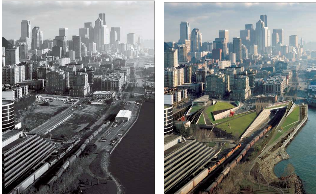
Figure 3.2. Site of the Olympic Sculpture Park Project before and after the construction. Source: Joan Busquets, ed., Olympic Sculpture Park for the Seattle Art Museum (Cambridge, Mass.: Harvard University Graduate School of Design, 2007), 26, 27.
