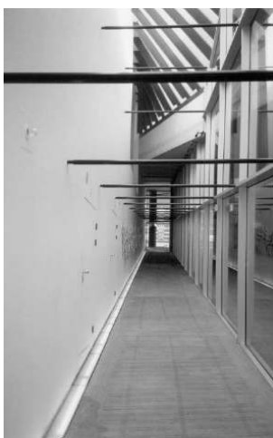
Figure 3.16. The interior ramp of the Kunsthall showing the continuity of materials between inside and outside. Source: Michel Moussette, “Do We Need a Canopy for Rain?": Interior-Exterior Relationships in the Kunsthall,” Architectural Research Quarterly 7 (2003): 280.
