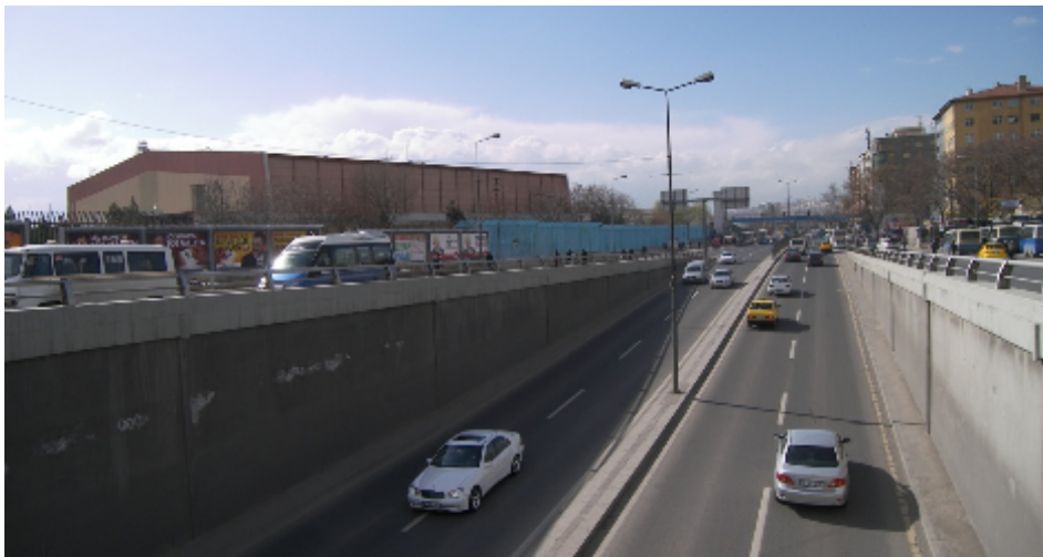
Fig. 4.13 The underpass on the North East edge of the Sports District Source: Photograph taken by Nezih Burak Bican on 26 th March 2009
