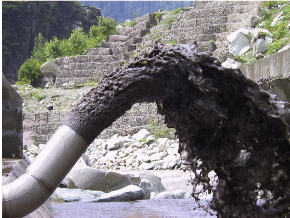
Figure 2.11 Silty sediments removed from pipeline
