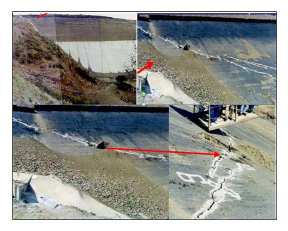
Figure 3.10 Cracking of face supporting zone at Xingó Dam (Souza, 2007)
