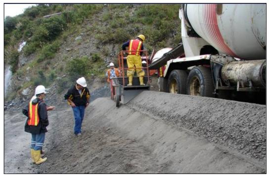
Figure 2.17 Site application of concrete curb casting (Orejuela, 2007)
