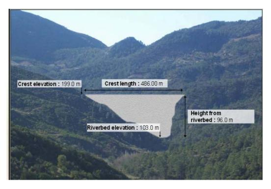
Figure 4.2 Proposed dam placement across Gökçeler River valley (Hidro Dizayn, 2007-b)
