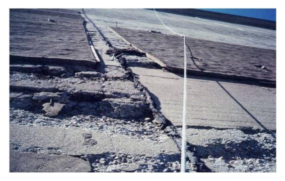
Figure 3.1 Deteriorated face slab of Salt Springs Dam (Scuero, 2007)
