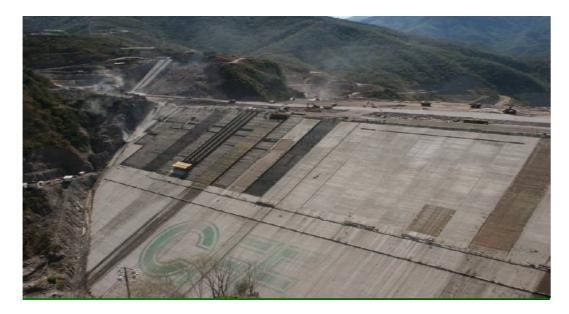
Figure 2.15 Site application of face slab construction (Marengo, 2007)
