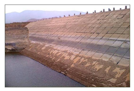
Figure 2.2 Traditional face slab of Caritaya-Presa Dam in Chile (Quezada, 2007)
