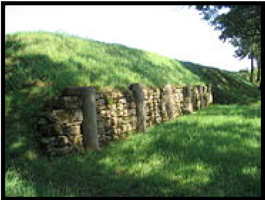
Figure 3.45 Reconstructed Kelheim-style rampart at the oppidum of Burgstall (Finsterlohr), Germany.
