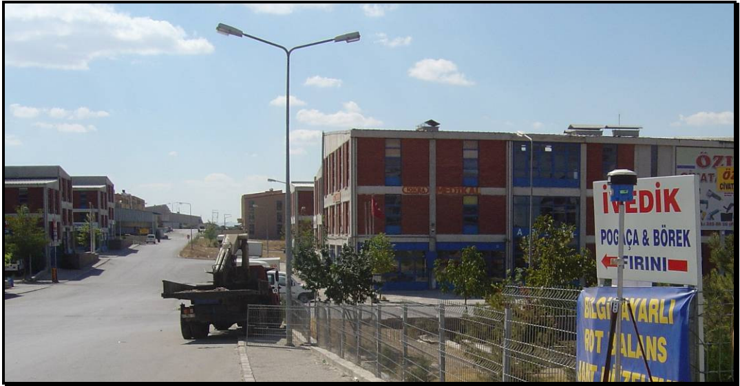
Figure A. 6. Photographs of rectangular shaped industrial buildings from the study area
