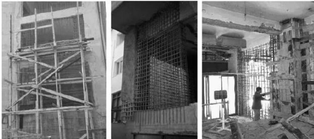
Figure 1.4 Typical cast in place infill panel
