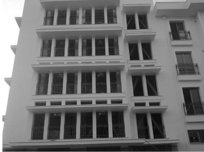
Figure 3.3 Office building under rehabilitation
