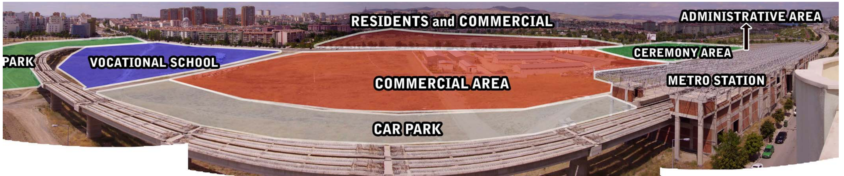
Figure 6-16 North View of the Central Area of Batkent
