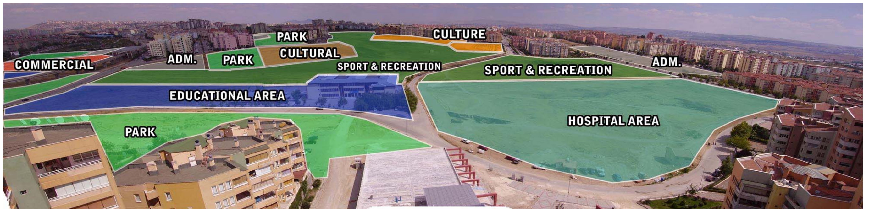
Figure 6-17 East View of the Central Area of Batkent
