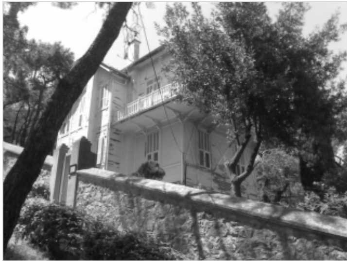
Figure 4. 14: Entrance to the garden source: (Sevil Enginsoy Ekinci, August 2009)
