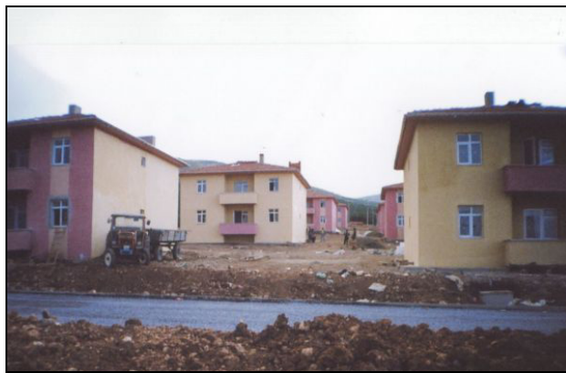
Figure 4.8. Earthquake Houses Constructed by the State (TOKI) in Afyon (Inaz) after the ZDS System (Source: Afyon Haber 2008)
