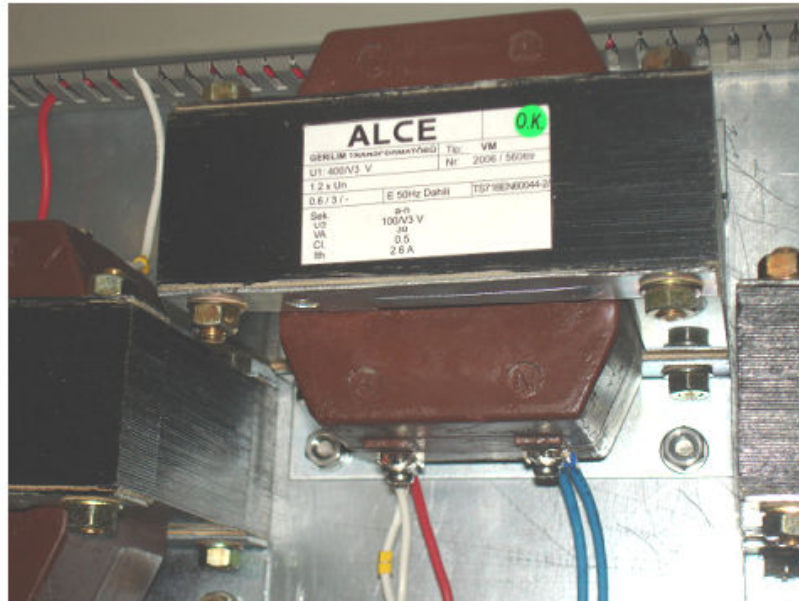
Figure 4.31 0.5P Class Voltage Transformer
