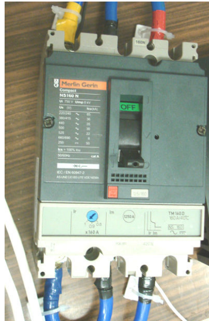
Figure 4.26 Circuit Breaker
