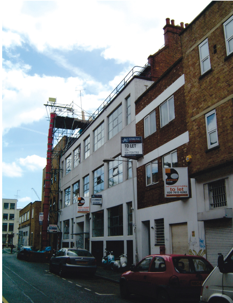
Figure 28: Erection of a Wind Turbine in Conservation Area (Hackney Council 2002:4)
