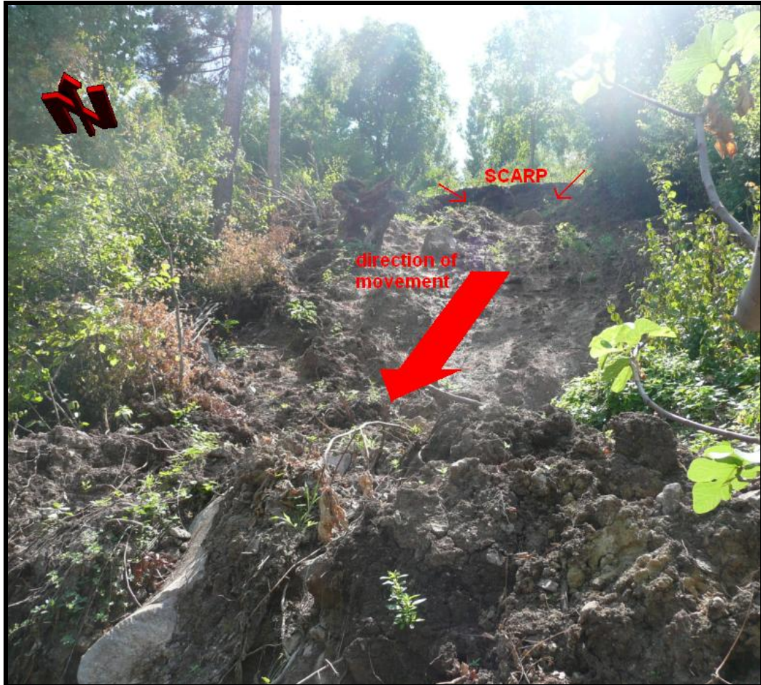
Figure 3.7. The scarp of an active landslide. The photograph is taken from the point having coordinates of UTM Zone 37T, 4495175N and 327627E.
