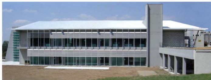
**Figure 3.2** South façade of the MATPUM Building showing the fixed sun breakers
