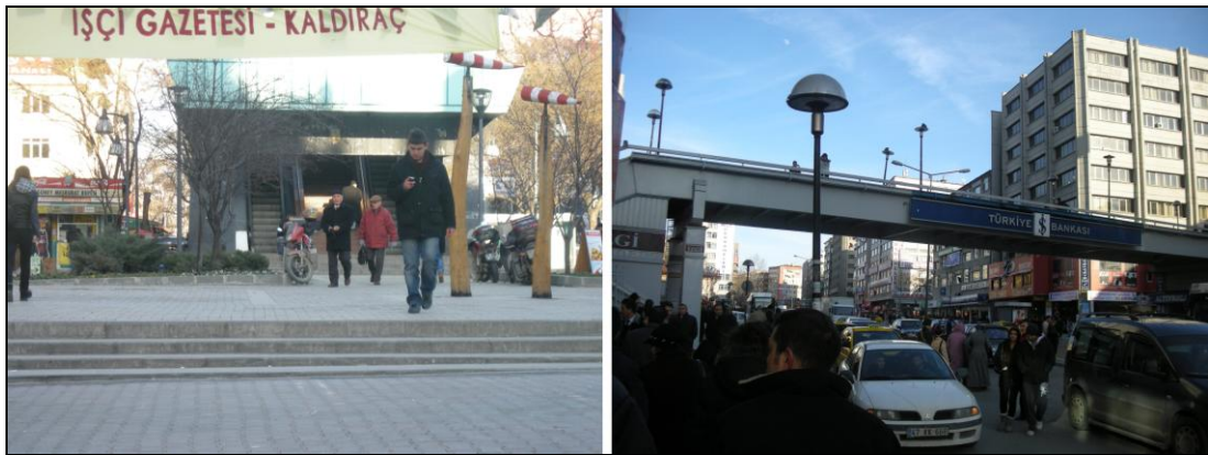
Figure 11: Appearances of pedestrian overpasses in Sakarya Precinct and Ziya Gökalp Boulevard (Source: Personal archive)
