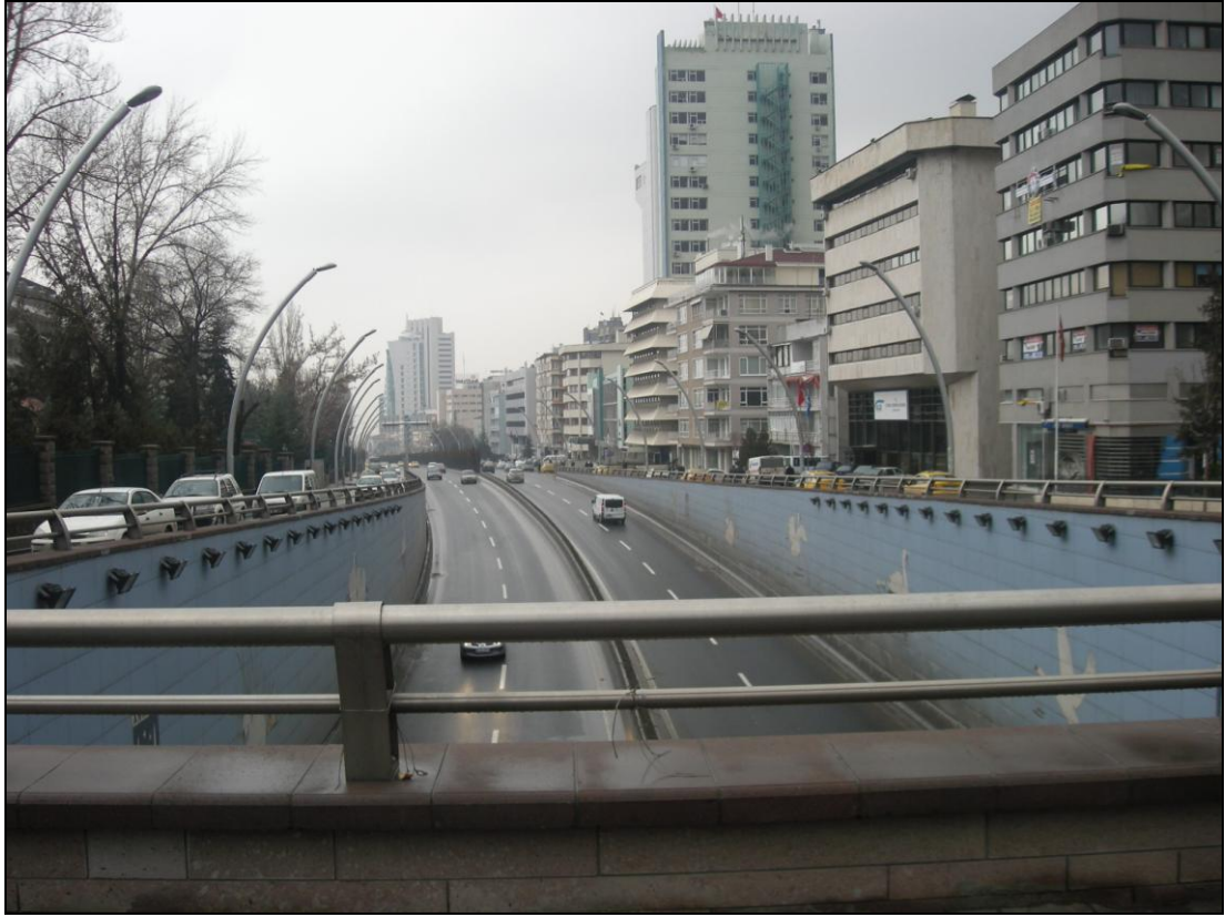
Figure 13: Appearance from Kuğulu Underpasses (Source: Personal archive)
