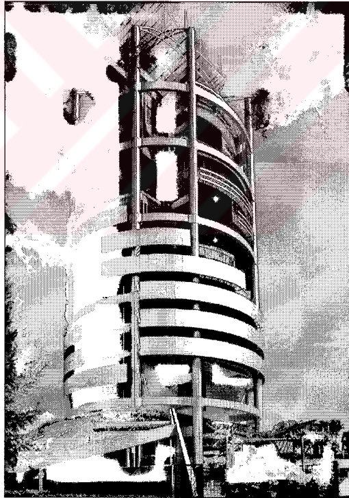
Photo 3-2. Menara Mesiniaga, in Kuala Lumpur, Malaysia, its analysis is on Figure 3-12.
