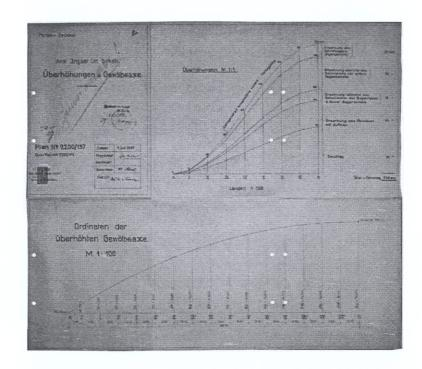
**Figure 4.27** Drawings of the reinforced concrete arch of the Pertek Bridge, by Prof. Mörsch, in 7.07.1937 Source: State National Archives-Republican Archives, Binder no: 2319
