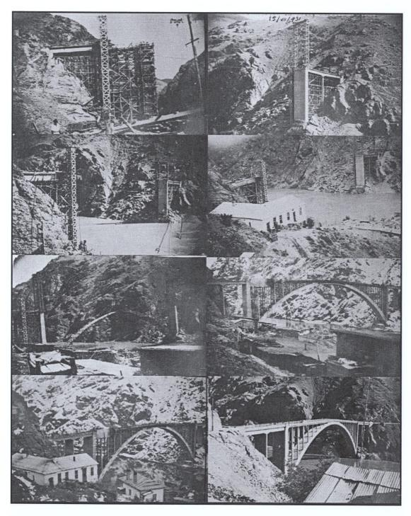
**Figure 4.22** Photographs of construction process of Kömürhan Bridge between 1930 and 1932. From left to right, up to down: 1. construction of neighboring spans, 2. construction of temporary towers, 3 and 4. cables between two towers, 5. suspension of the centering, 6 and 7. pouring the deck and protection of concrete against freeze, and 8. the completed bridge. Source: Unclassified documents from the State National Archives-Republican Archives, KGM Fund, Binder no: 16041
