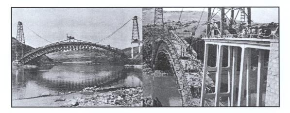
Figure 4.25 Pertek Bridge underconstruction. Photographs showing suspention type centering as in case of Kömürhan and mechanism especially built for concrete pouring, circa 1938. Source: KGM Archieves and available on 22.2.2008 at http://wowturkey.com/forum/viewtopic.php?t=88872
