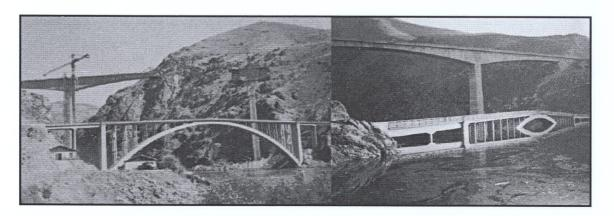
Figure 4.24 Photographs of old and new Kömürhan bridges together. Right: During construction (1984), Left: During submerging (1987). Source: KGM Archives, off-track bridge files, region 8.
