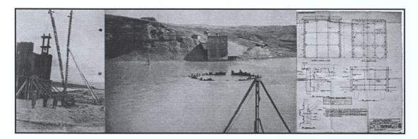
Figure B.10 From right to left: Pile-plank drawings of Cizre Bridge, pile-plank foundation in water in Cizre Bridge, pile-plank sheets while driven into soil in Singeç Bridge construction. Sources: Unclassified material from KGM Fund, Binder No.2367 and 2325, State National Archives of Turkey-Republican Archive, Ankara.
