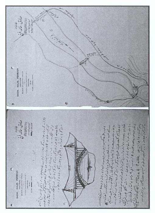
Figure 4.15 Pages from letter from SaFerHa to Nadir Bey, the Director of the Roads and Bridges Department, on 28.8.1928. Right: showing three possible locations, Left: sketch about the possible centering system for an RC arch bridge. Source: Unclassified documents from the State National Archives-Republican Archives, KGM Fund, Binder no: 16041
