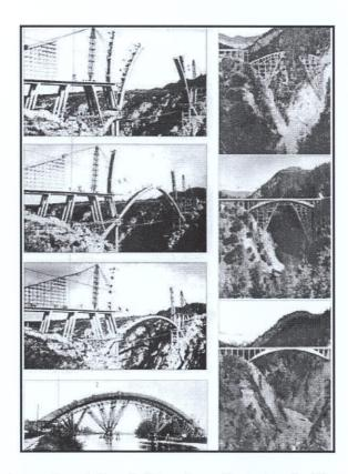
**Figure B.11** Various types of centering. Left top three: Centering for River Storms Bridge, South Africa; left bottom: centering for St. Pierre de Vauray, France; right: centering for Salgina-Tobel Bridge-Switzerland. Sources: Troyano, F., "Bridge Engineering", Thomas Telford Publishing, 2003, pp.170, 291, and 333.
