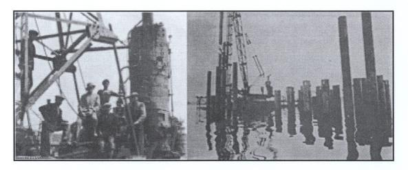
**Figure 3.12** The steamed pile-driving machine of SaFerHa on piling works in construction of Gazi Bridge in 1930. Sources right to left: Erer, T., "Boğaziçi Köprüsü", Boğaziçi Yayınevi, Istanbul,1973, p.223 and Available on 10.10.2009 at www.stfa.com
