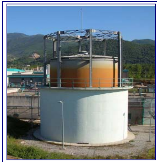
Figure 2.21 Floating Top Biogas Holder
