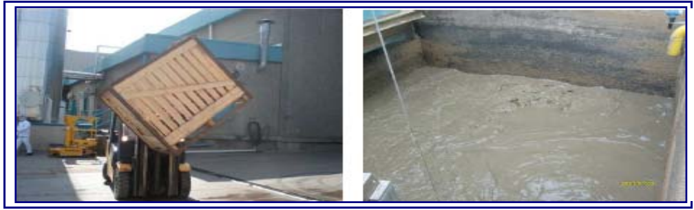
Figure 2.13 Forklift carrying Organic waste Figure 2.14 Equalization basin with mixer
