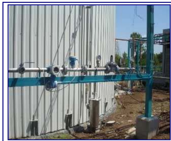
Figure 2.22 Biogas measurement and monitoring instruments
