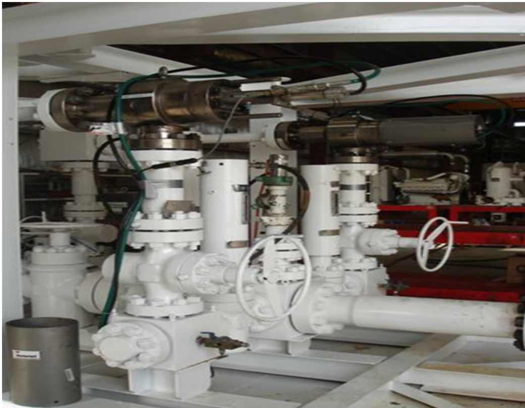
Figure 59 Semi-Automatic Choke Manifold System 41
