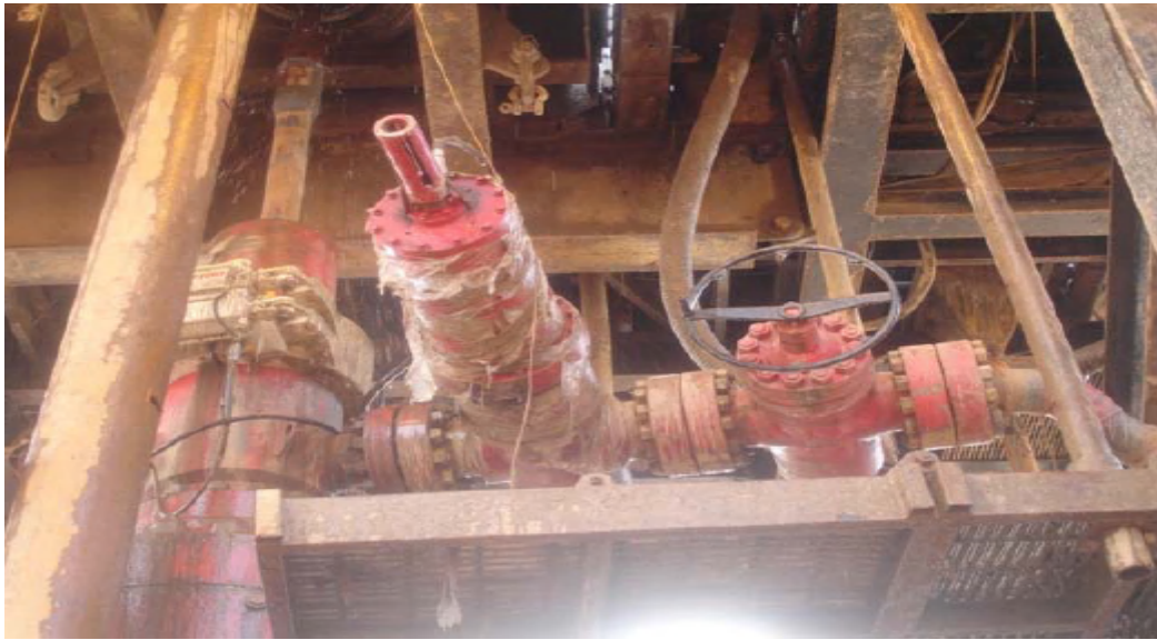
Figure 31 Photo of Rig Gas Booster 15
