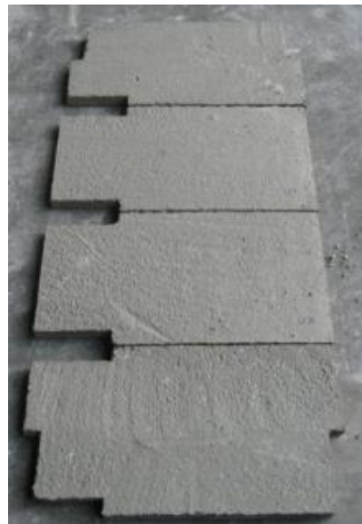
Figure 4.21 General view of the precast concrete panels.
