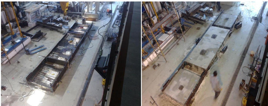
Figure 4.5 General views of the foundation before and after pouring of concrete
