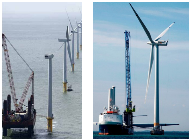
Figure 1.12 Cranes to install offshore turbines. 6
