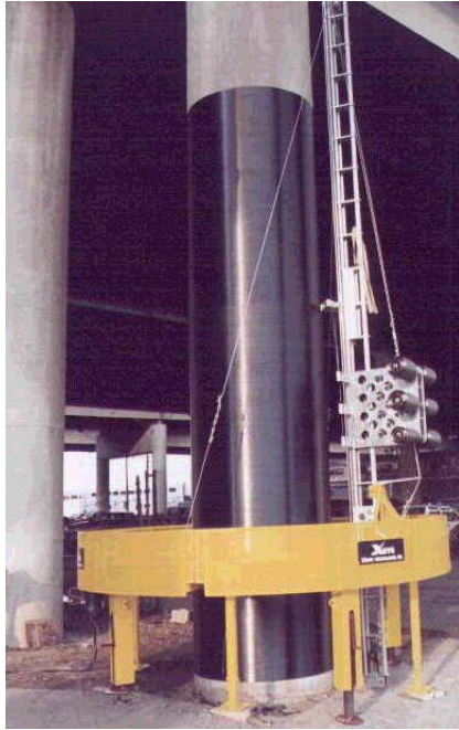
Figure 1.7 The ROBO-Wrapper I™. A freeway column retrofit filament winder. [8]
