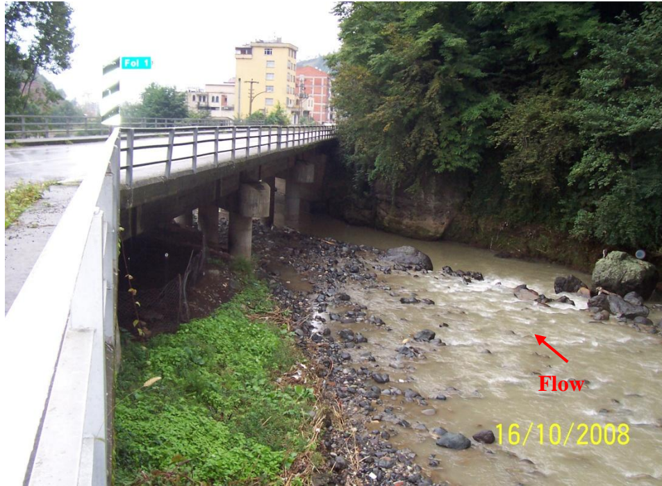
Figure 3.9 A view of the bridge site from its upstream
