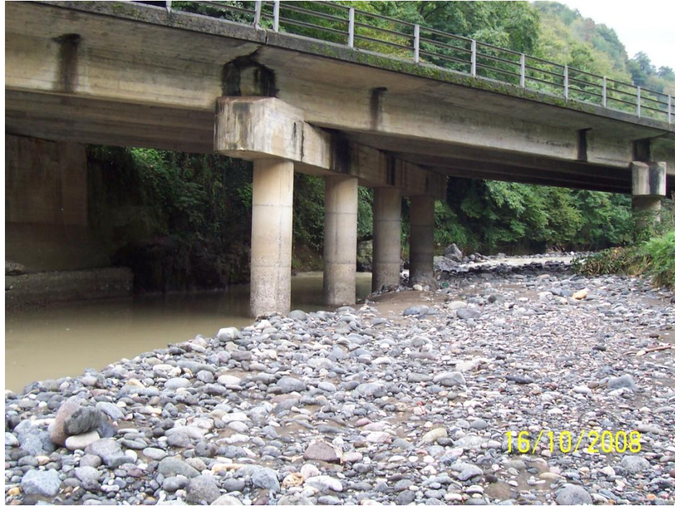
Figure 3.7 Bridge deck skewed to flow
