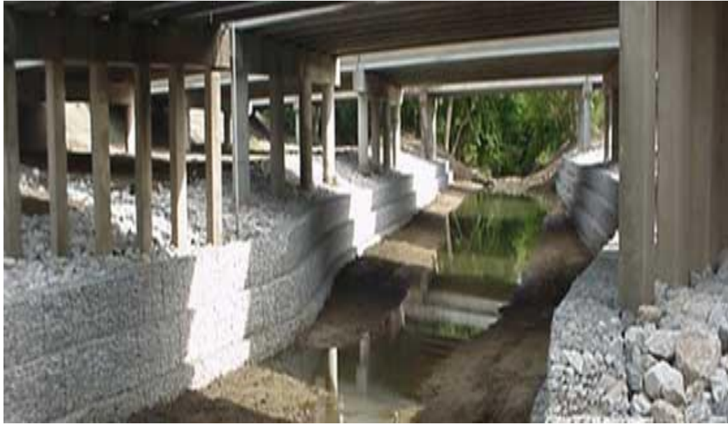
Figure 3.14 Use of gabion boxes around bridge piers (Red Star Wire Mesh Factory, 2006)
