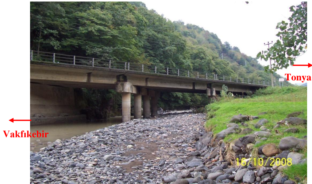
Figure 3.2 A view of the study bridge from downstream
