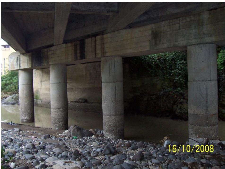
Figure 3.6 Right piers and abutment (Vakfikebir side)
