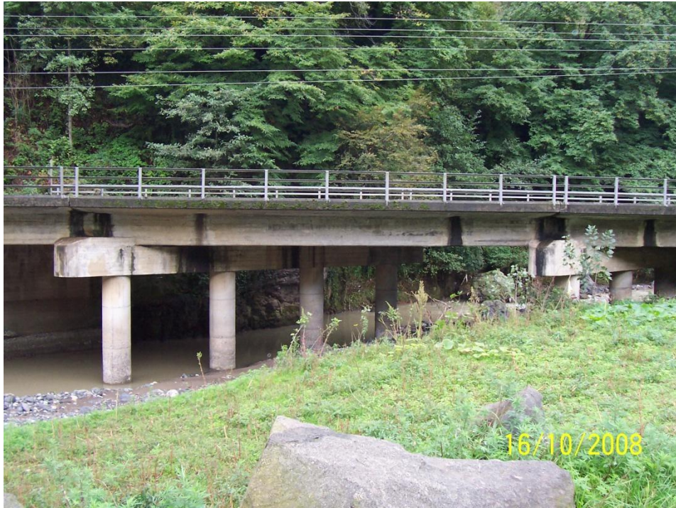
Figure 3.5 General view of Fol-1 Bridge
