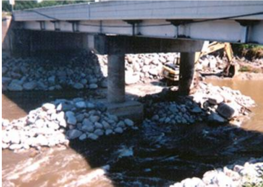
Figure 3.12 An application of riprap around bridge piers (Newsline, 2007)
