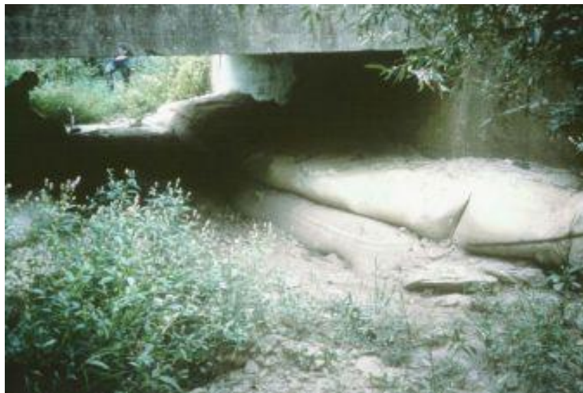
Figure 3.13 An application of grout filled bags around bridge abutment (Lagasse, 2002)
