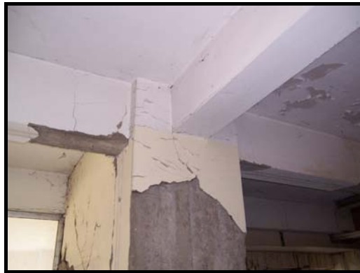
Figure 4.45 Interior joint between the ground story column-C6 and beams B7-B8-B17-B18 (Bolu)
