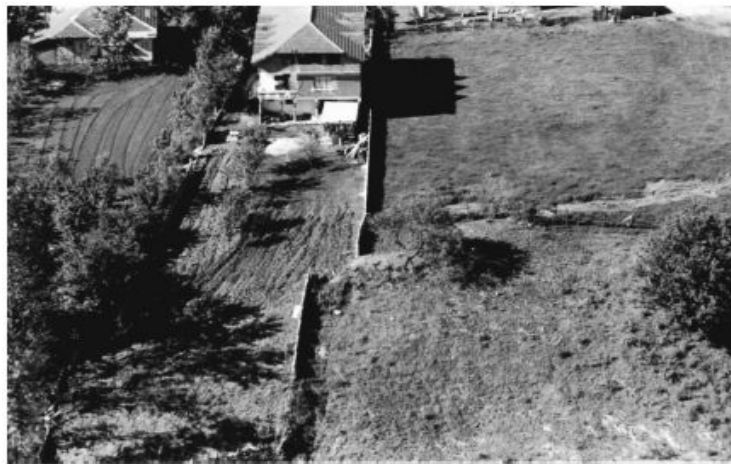
Figure 4.14 Offset (4.5m) garden fences around Çınarlı village (Akyüz et al., 2002)
