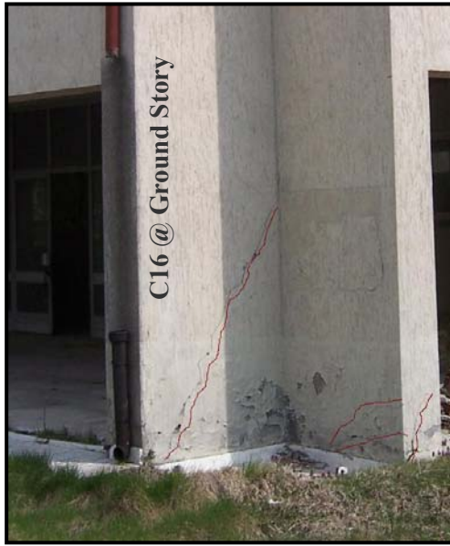
Figure 4.31 Shear cracks in the ground story column-C16 (Bolu)
