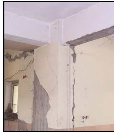
Figure 4.46 Interior joint between the ground story column-C7 and beams B8-B9-B20-B21 (Bolu)
