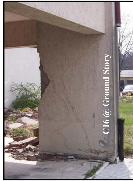
Figure 4.31 Shear cracks in the ground story column-C16 (Bolu)
